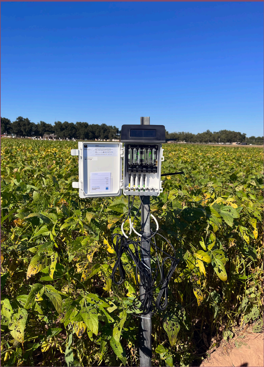
A soil moisture sensor installed in a field at the AgCenter Red River Research Station measures the status of fields used in Xi Zhang’s research. Photo by Xi Zhang
